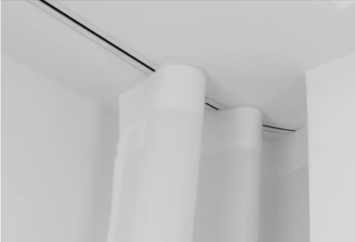
Trackrim® Curved Section finished installation.
